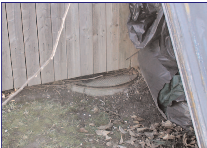
Example of encroachment onto Authority’s easement. Precious time is lost removing obstacles to manholes and sewer lines. Add snow and the manhole becomes very difficult to locate when there is a sewer backup.
